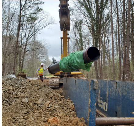
West Fork 12-Mile Creek Interceptor Construction Phase Services, Union County
