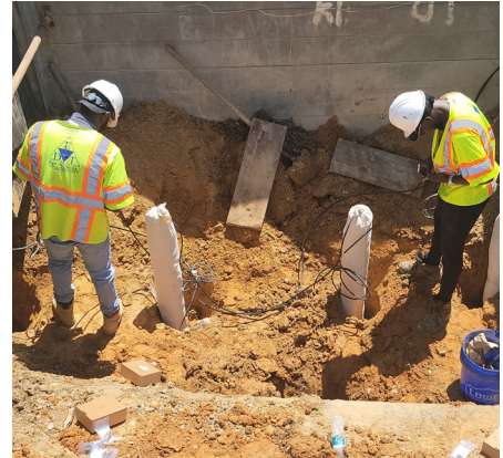
DC Water Anode Installation, Washington DC
