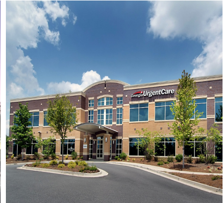
Alpharetta Medical Office Building
