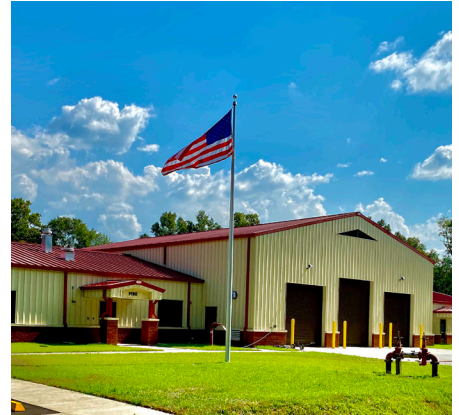
Satsuma Public Safety Building
